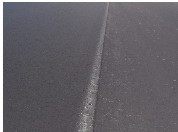
Figure 1.1-2 – Completed longitudinal joint with adhesive at Minnesota TH 100 during 2015 construction.
