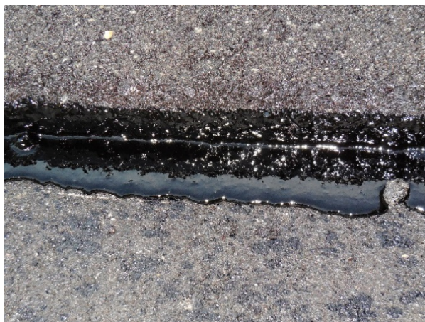
Figure 1.1-1 – Longitudinal joint with adhesive mastic at Minnesota TH 100 during 2015 construction.
